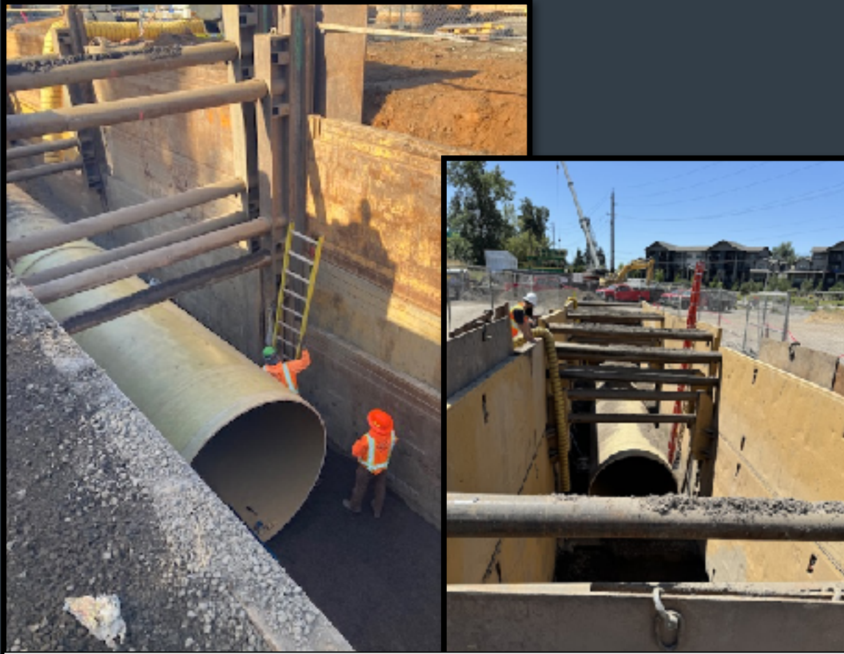
Open Cut Construction
